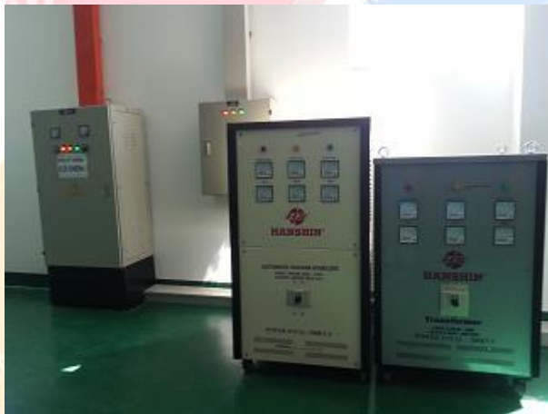
Hanshin transformer – Input : 3 phase 380V – Output : 3 phase 200V Biến thế Hanshin – 3 pha
