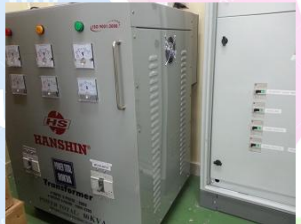
Hanshin transformer – Input : 3 phase 380V – Output : 3 phase 200V Biến thế Hanshin – 3 pha
