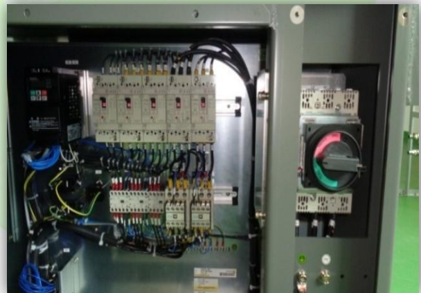
Power supply for machine – 3 phase 380V / 3phase 200V ( Japan machine )
