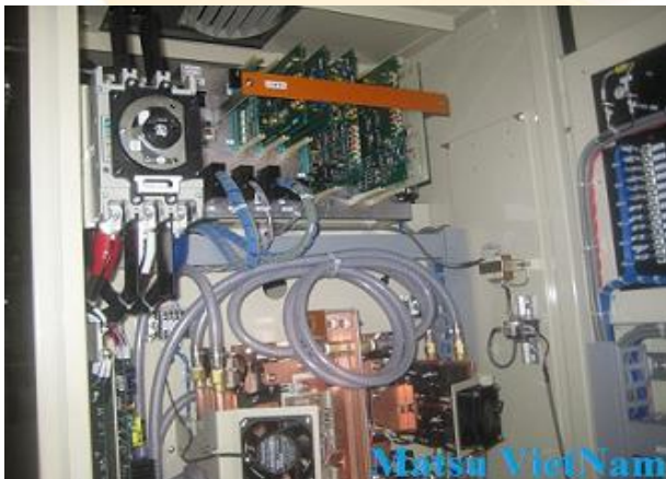
Power supply for machine – 3 phase 380V / 3phase 200V ( Japan machine )
